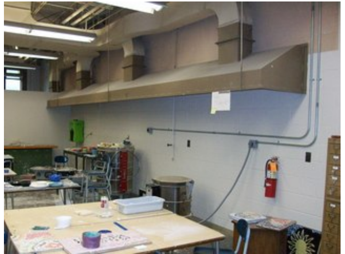
Art Kiln And Exhaust Hood
