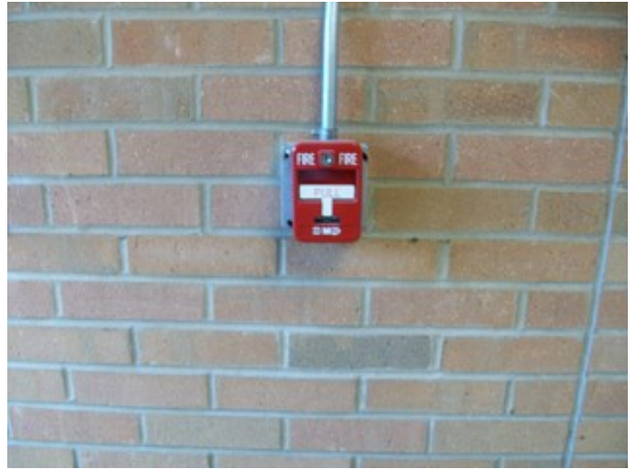
Fire Alarm Pull Station
