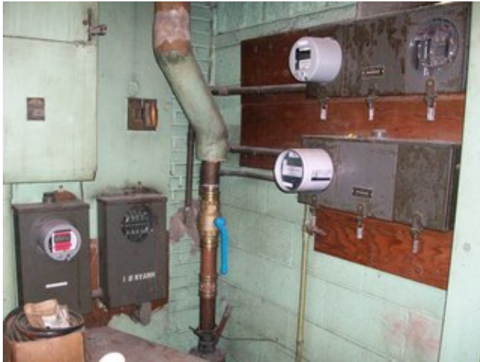
Domestic Water Piping
