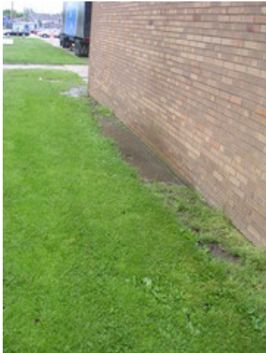
Poor grading at foundation.
