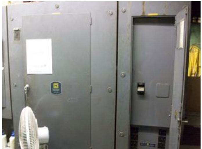
Main Distribution Panelboard
