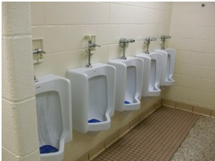
Toilet room fixtures
