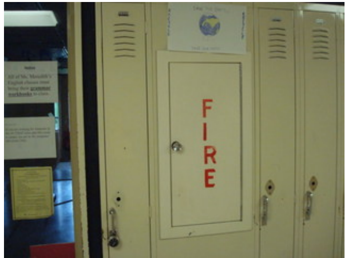
Fire extinguisher cabinet
