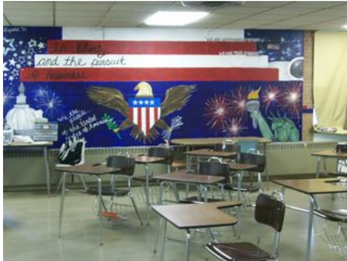
Baseboard Heating Panel
