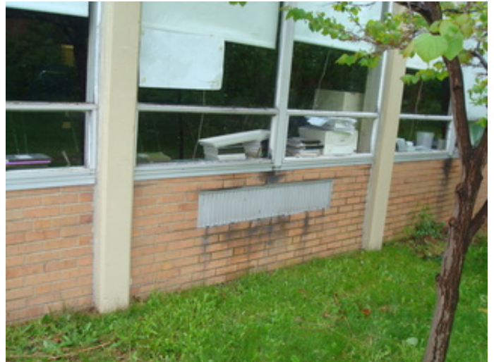
Deteriorated lower lintel at 1958 Original Construction
