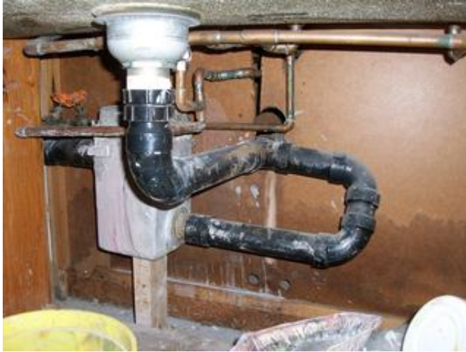
Sanitary piping below sink
