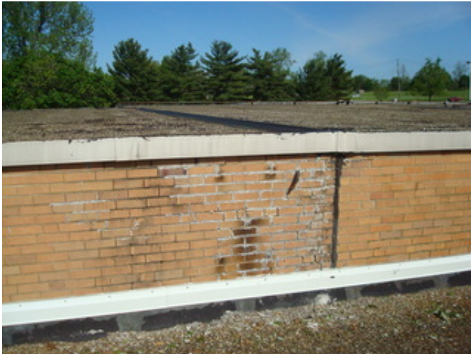
Water-damaged wall area at expansion joint at 1958 Original Construction
