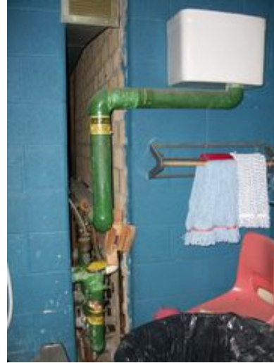
Sanitary drainage Piping in chase
