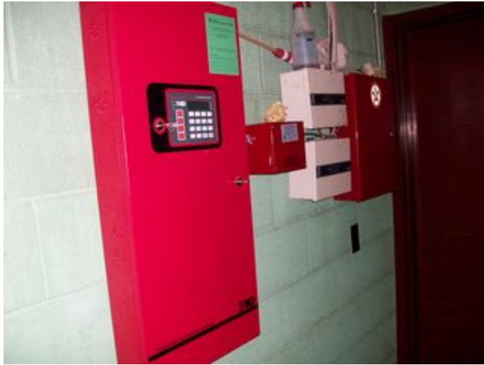
Fire Alarm Panel
