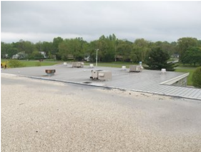
Roof Top Air Conditioners
