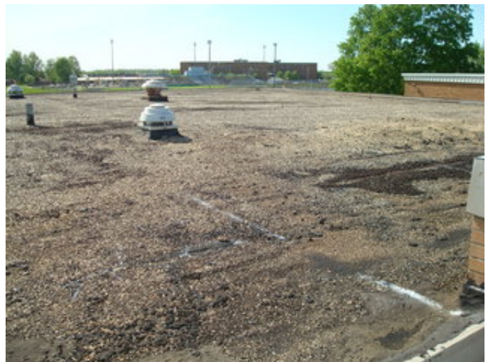
Built-up roofing over vocational area in 1967 Addition
