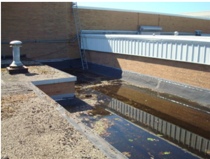
Ponding on 1958 Original Construction and roof ladder
