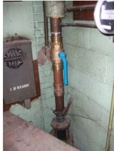
Domestic water piping
