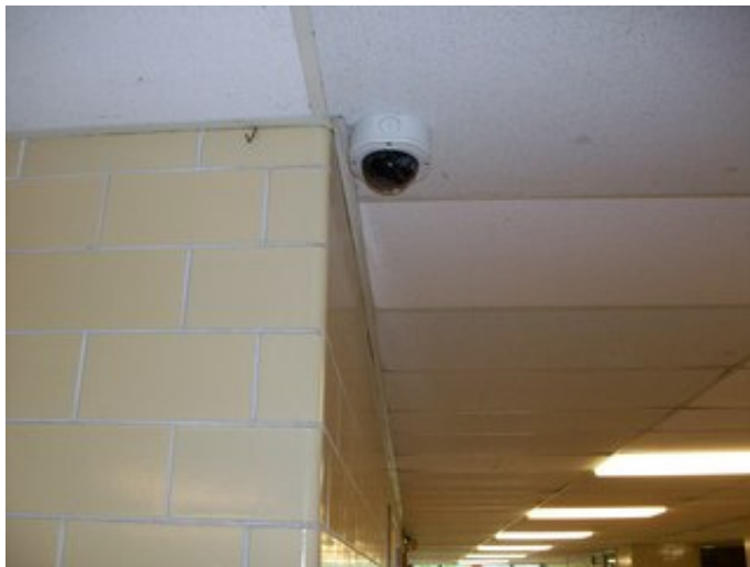
Ceiling Mounted Security Camera
