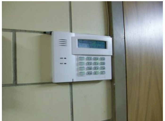
Wall Mounted Security Panel
