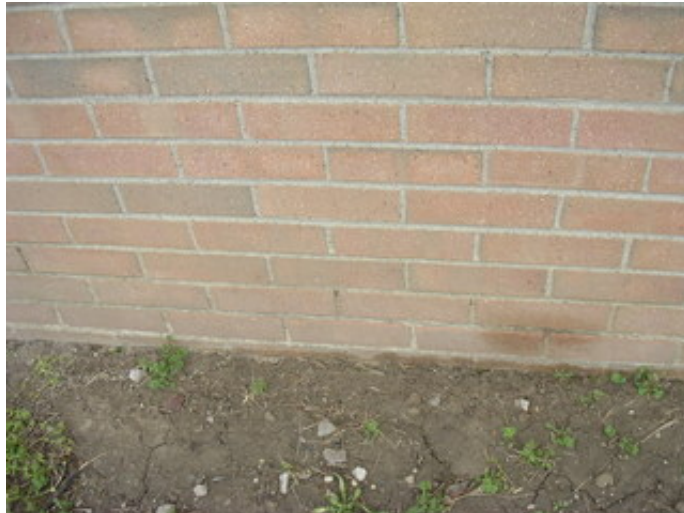
Typical foundation condition.
