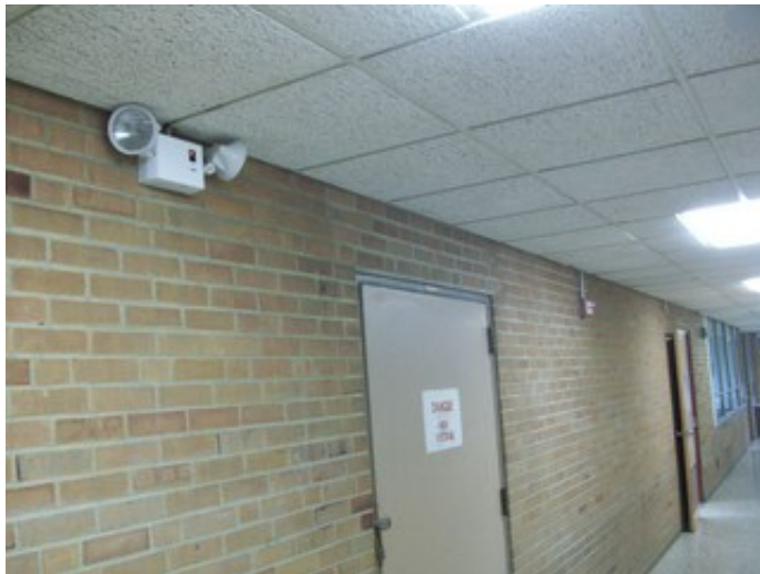
Wall Mounted Emergency Lighting
