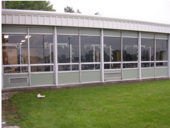
Typical aluminum storefront system.
