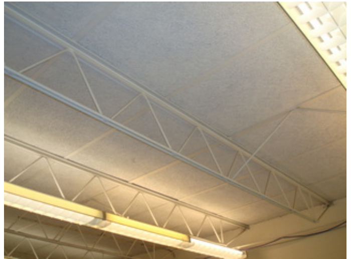
Roof structure exposed in classrooms
