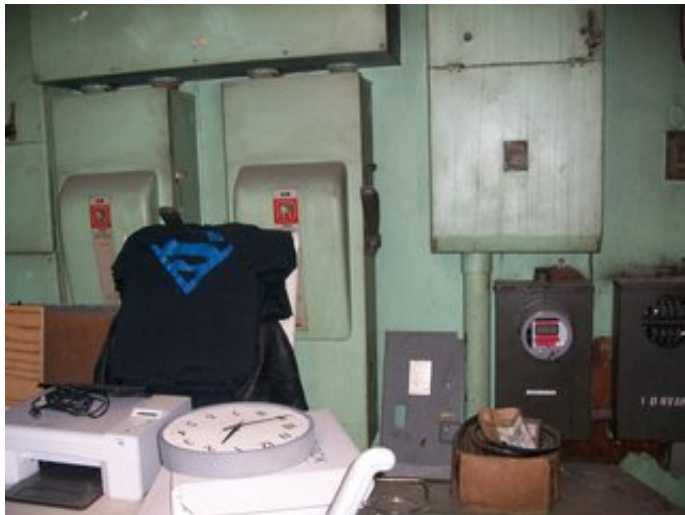
Typical Main Disconnect Switches
